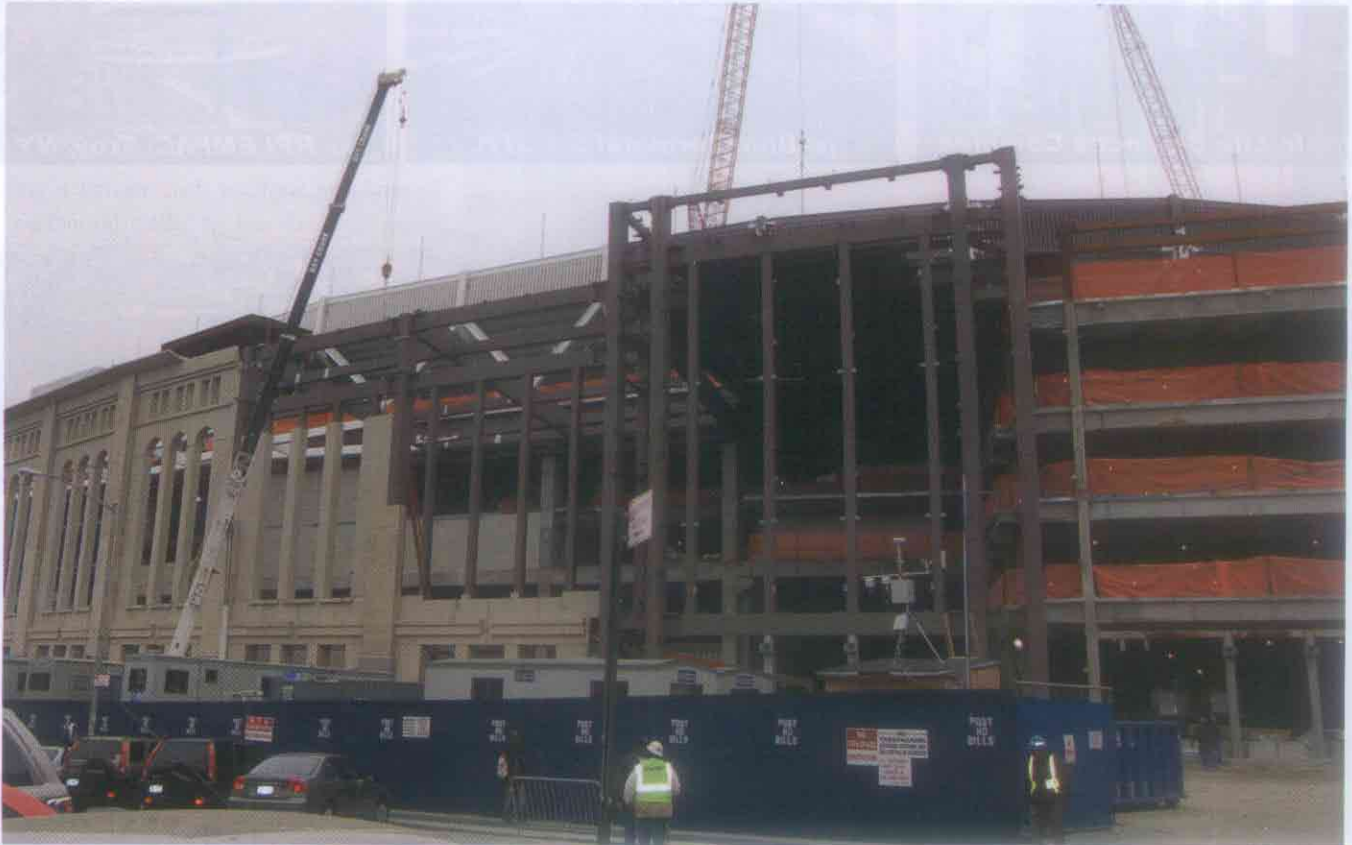
The new Yankee Stadium, which, like Citi Field, was designed by HOK Sport of St. Louis, is intended to resemble the original "House that Ruth Built" which opened in 1923. The exterior will feature the same type of limestone and granite used in the original, which was remodeled in the 1970s. Photo by Andrew Wright.
